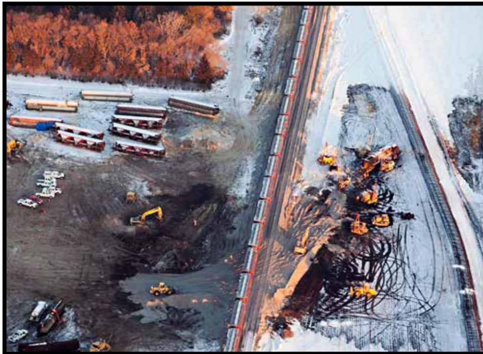
Figure 4 Casselton, North Dakota Oil Train Derailment
